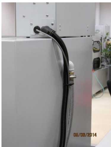
Assembly of cable
